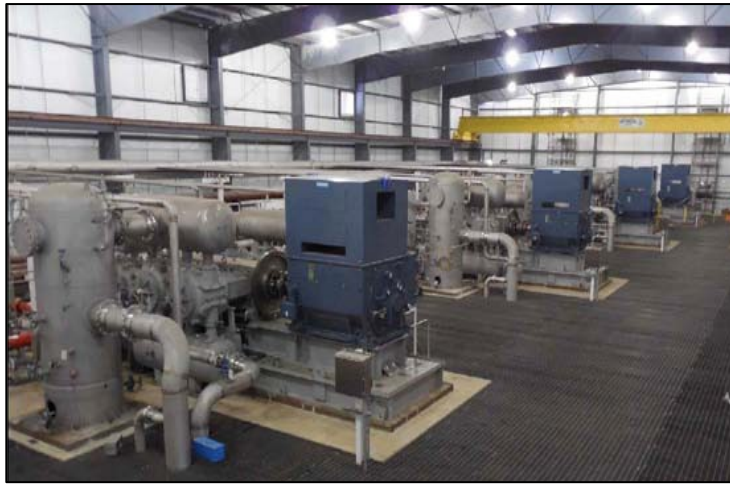
Four Compressor Train
