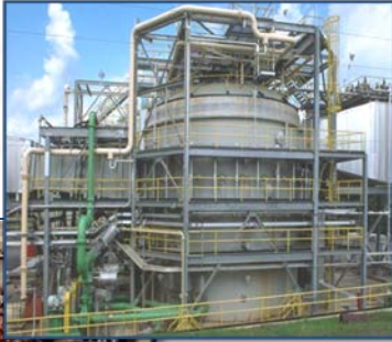
Flue Gas Desulfurization (FGD) Scrubbers
