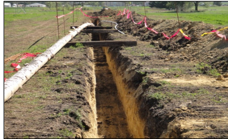
8" High Pressure transmission Line
